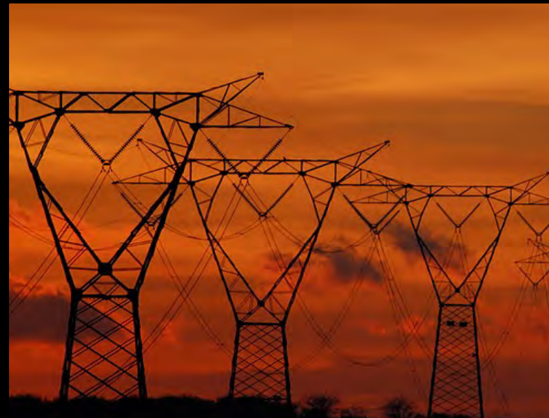
Power St. Enel Saragozza
